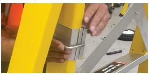
Secure with Nuts: Wind the nuts onto the U-bolt and tighten them using torque wrench 9Nm to secure the bracket in place.
