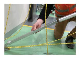
• Tension the tether system. The ladder should be rigidly secured to the structure at this point.
