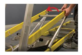
Latch the platform hooks onto the ladder rung
